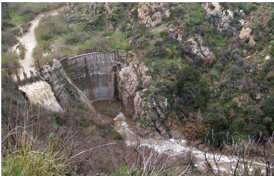
Rindge Dam on Malibu Creek, completely filled with sediment, is slated for removal so that Steelhead trout can access Upper Malibu Creek.
