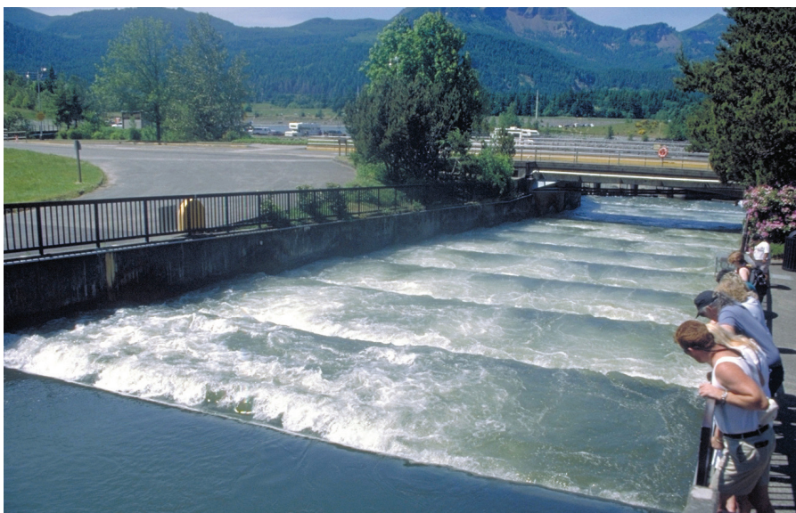
A fish ladder on the Columbia River helps fish on their journey upstream, but is not as successful in helping fish on their way down.
